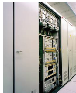
Original CJR01 Cabinet with SIMADYN and ISKAMATIK
