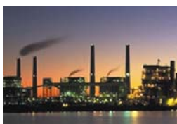
Parish, USA Low Loss Start Minimum Load Reduction Fast Ramp
