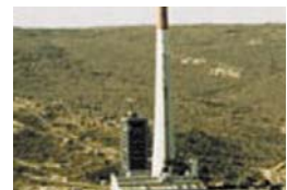
Plomin, Croatia Fast Start Temperature Optimizer Fast Ramp Frequency Control
