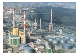
Simmering, Austria Low Loss Start Temperature Optimizer Low Stress Dispatch Control
