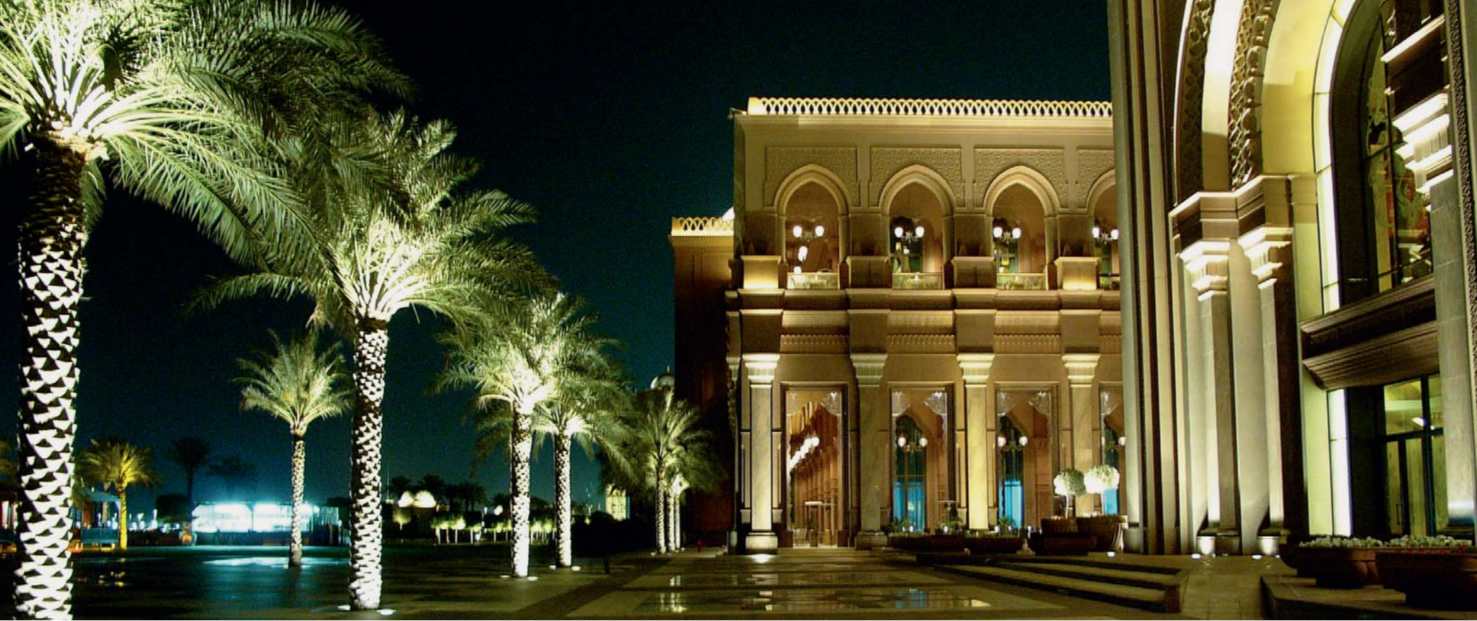
The rear exterior of the Emirates Palace Hotel. Siemens provided the medium-voltage switchgear technology for the impressive traditional structure.
