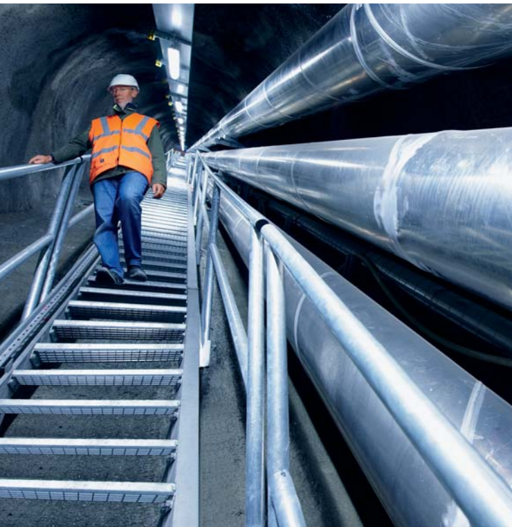
A view of the GIL shaft of Limberg II, Kaprun, Austria. The shaft gradient is 42 degrees.
