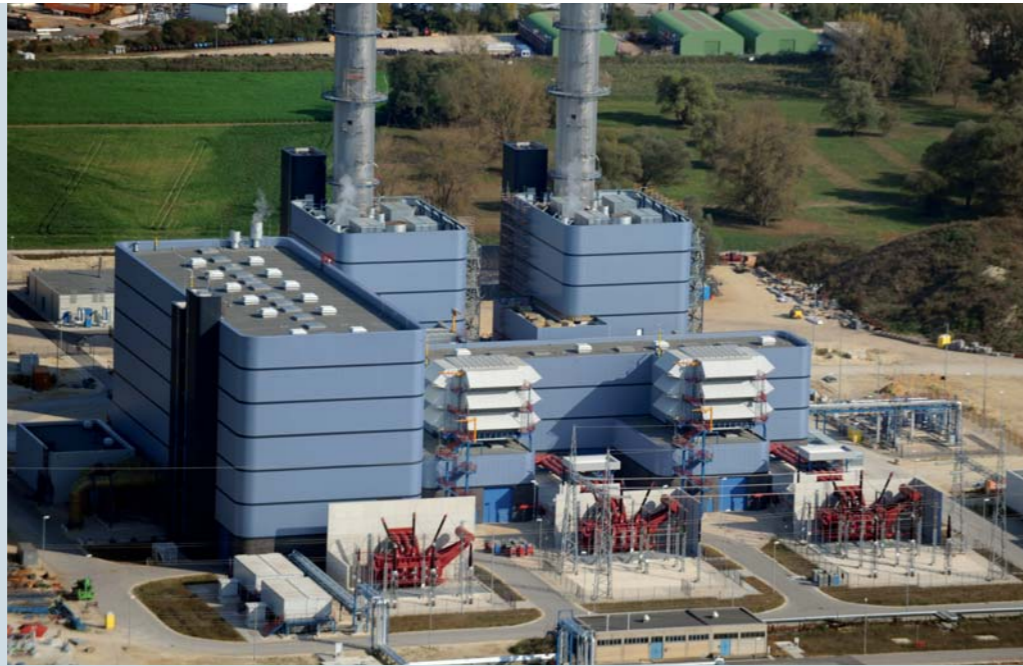
The new Irsching 5 combined-cycle power plant near Ingolstadt, Germany: a quick gust of backup power when the wind doesn't blow.
