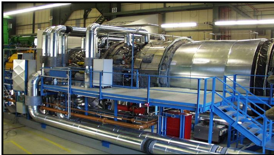
Figure 12. Berlin Test Bed for Full Load Engine Testing
