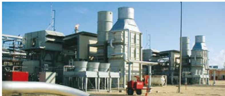
The first two SGT-700 mechanical drive onshore units were delivered to an NGL (natural gas liquids) plant in Egypt.
