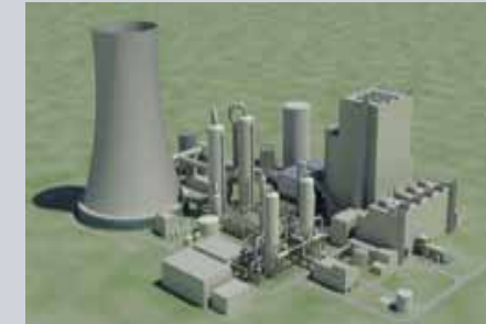
Post-Combustion carbon capture plant design
