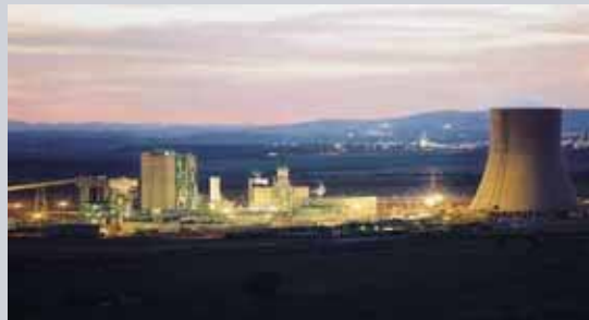
Siemens IGCC technology applied in Puertollano (E)
