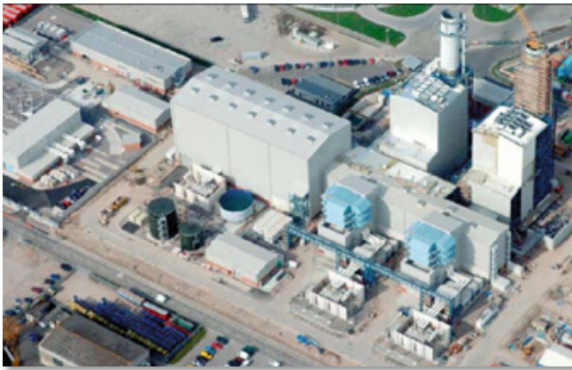
Figure 9. The 840 MW Marchwood combined cycle plant (SCC5-4000F MS)
