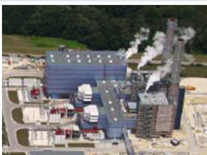
Figure 7. The 860 MW Irsching 5 combined cycle plant (SCC5-4000F 2+1)
