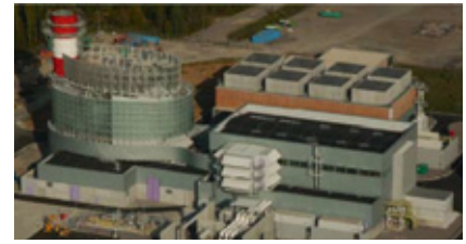
Figure 6. The 430 MW Pont sur Sambre combined cycle plant (SCC5-4000F 1S)
