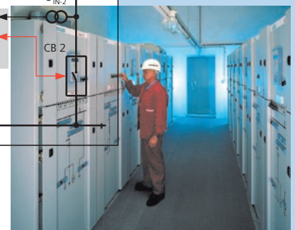
Fig. 2: Siemens High-Speed Busbar Transfer System Type AUE ensures high availability of power for important electrical consumers.
