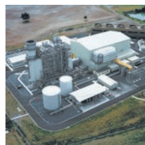
Fig. 8: Combined cycle power plant
