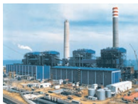
Fig. 7: Steam power plant
