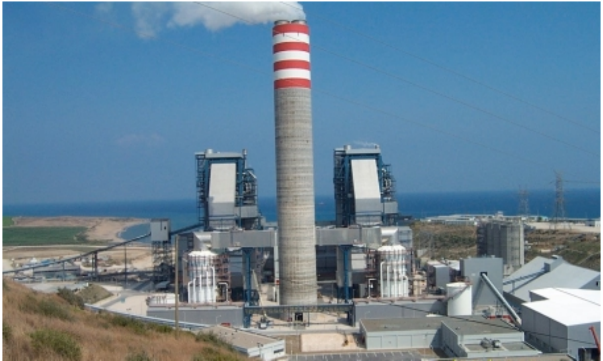
This picture indicates an overview of the Power Station from the north.
