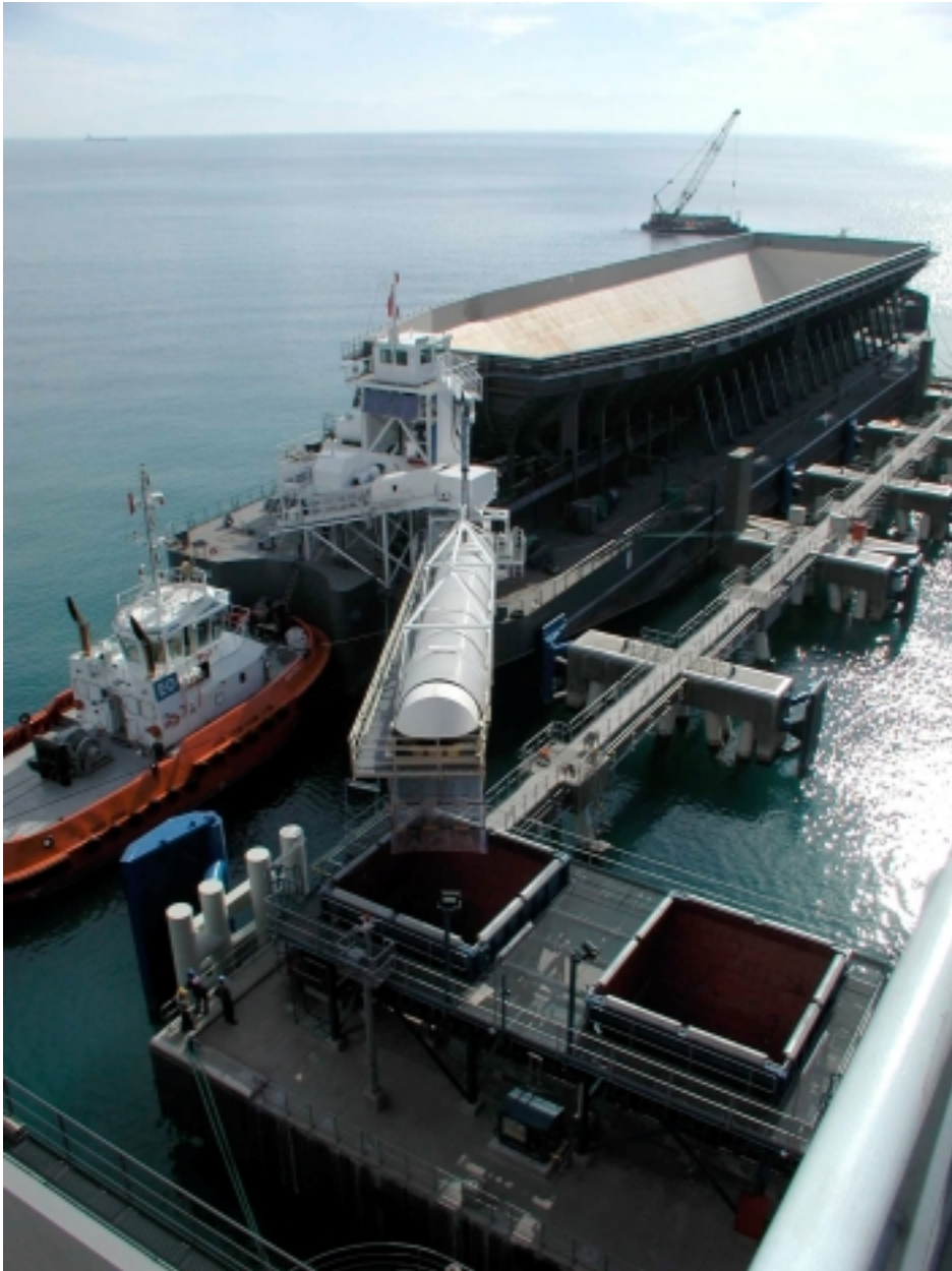
Barge Unloading at the Jetty
