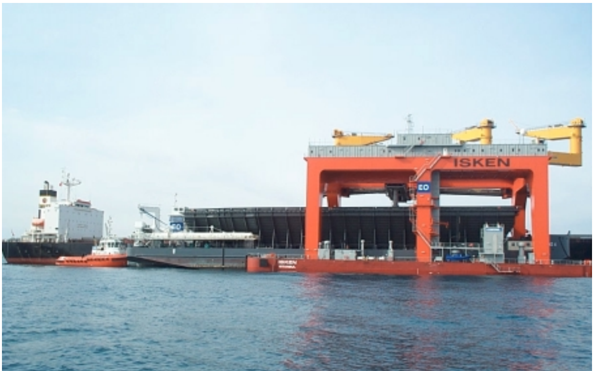
Coal Unloading by Transshipper Equipment
