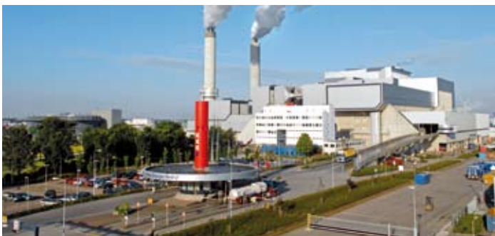
Amsterdam, Netherlands: AEB's waste fired power plant uses a 74 MW(e) extraction condensing turbine in reheat configuration.
