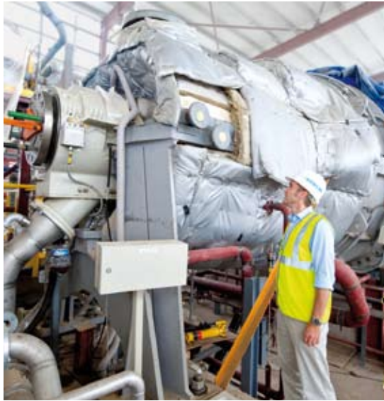
SST-700 IP turbine at the Solnova 1 CSP plant near Sanlúcar la Mayor, Spain.
