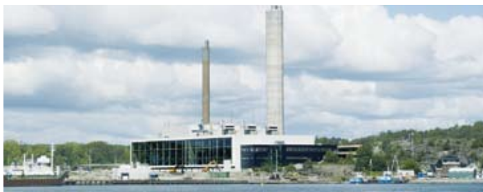
The Rya CHP plant in Gothenburg, Sweden, is powered by three SGT-800 gas turbines and one 137 MW SST-900 steam turbine.
