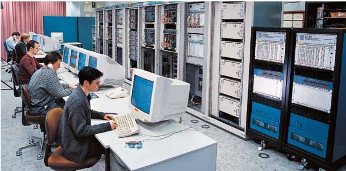
Fig. 5-2: Example for a Functional Performance Test Set-Up
