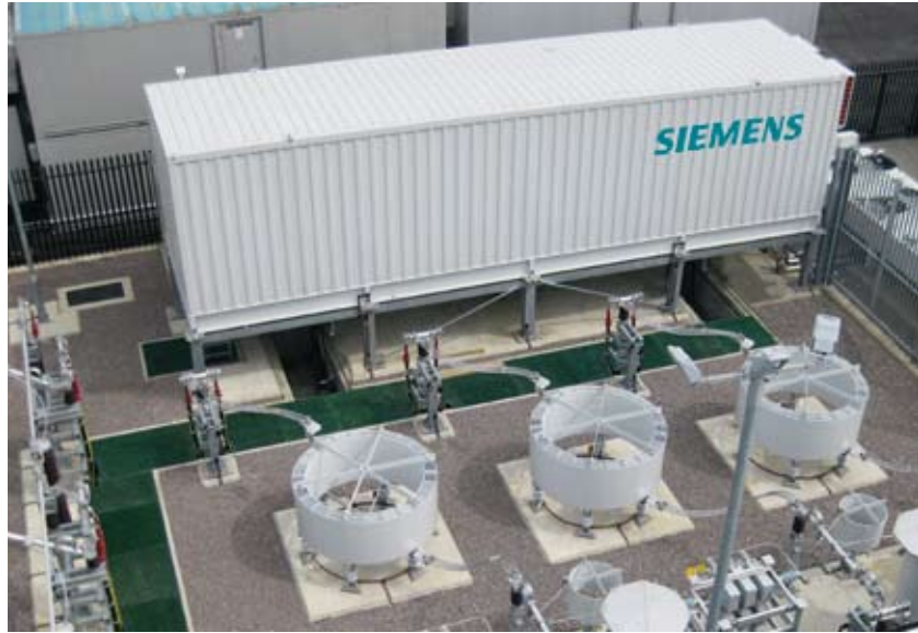
SVC PLUS from Siemens stabilizes power grids, helps increase the capacity of existing AC networks, and ensures grid code compliance.
