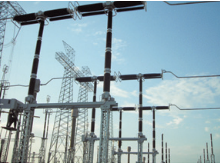
One-and-half breaker arrangement 800 kV, 2 BB
