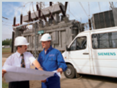
Reliable energy supply and optimized capital utilisation due to innovative condition monitoring solutions and tailored service contracts and service projects.
