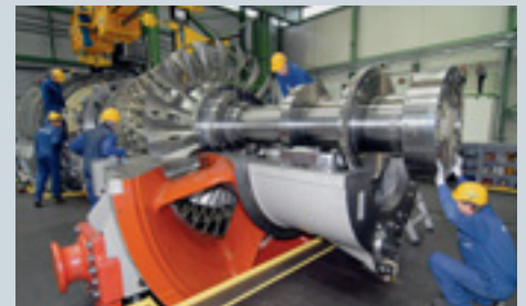
Real teamwork: Everyone pulls together to help install a turbine rotor.
