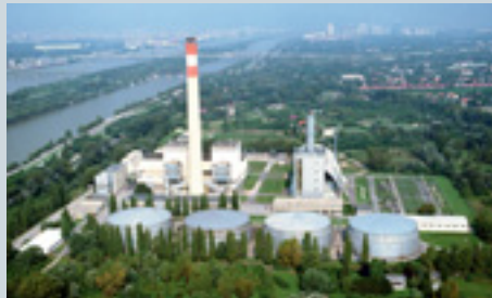
Siemens' customized services can also include the complete operation of the power plant.
