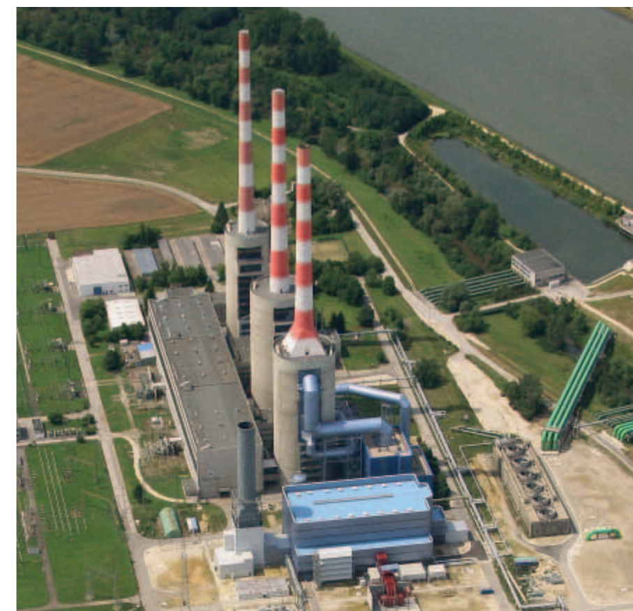
Author Craig Morris visits the world's largest gas turbine in an open-cycle power plant. The turbine is already installed and is currently waiting for the steam turbine and balance of plant to be added downstream.
