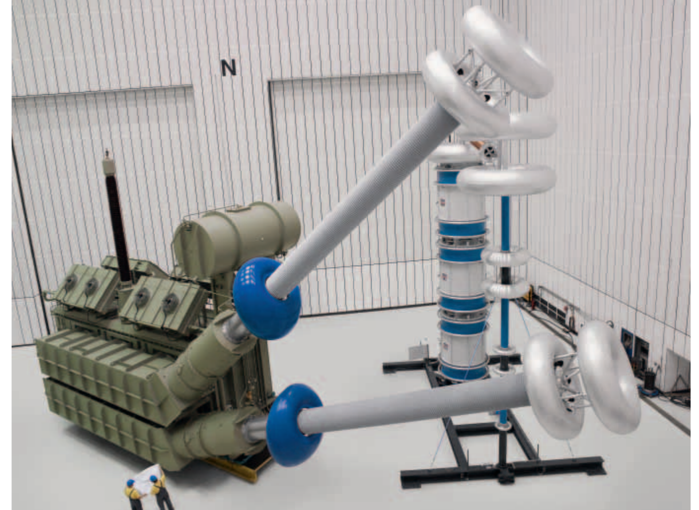
Behemoths in action – as this “snapshot” from UHV DC transformer shows, the equipment is the size of the entire building. Those are not ants in the pictures, they are people.
