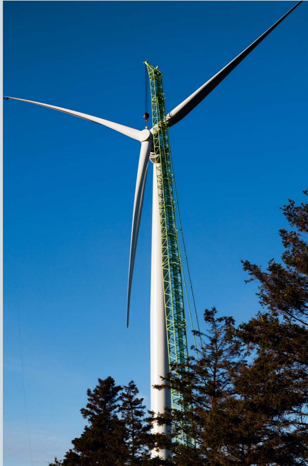
The new SWT-3.0-101 machine being erected in Drantum, near Brande, Denmark.
