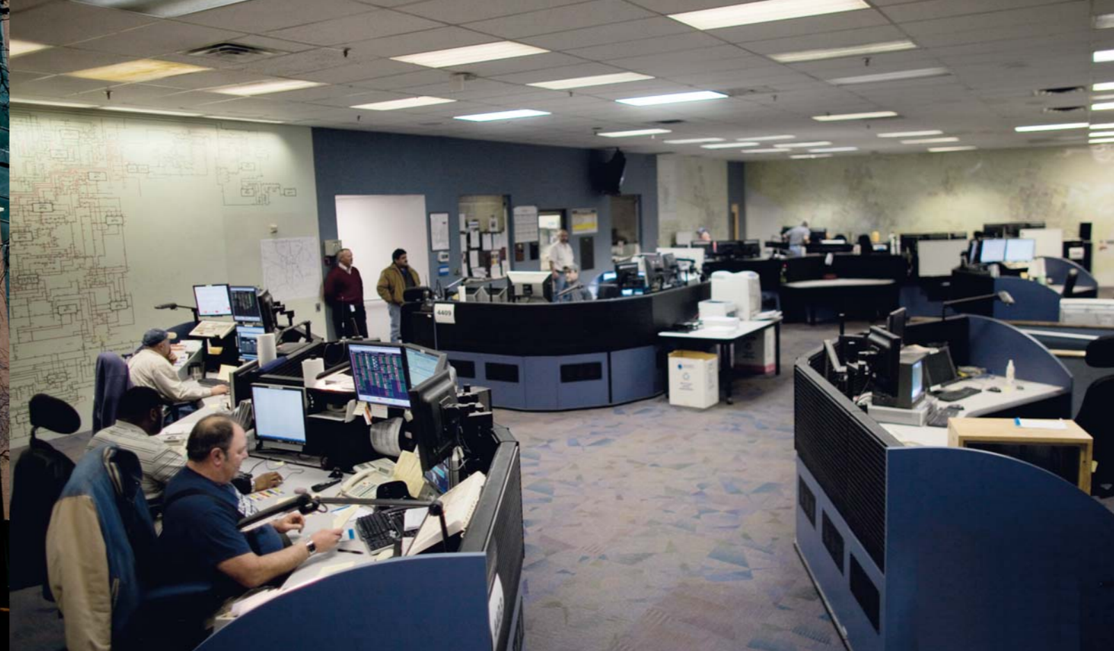
The control room: Smart grid management means calm in the eye of the storm.
