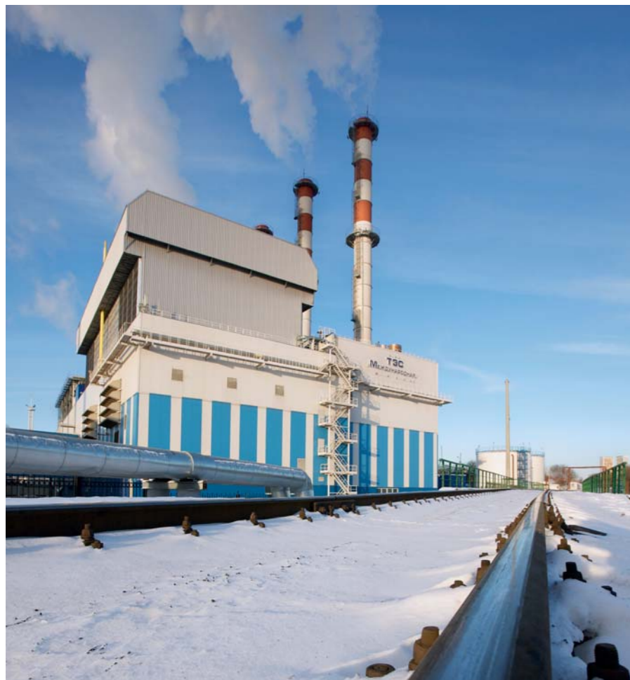
The HRSG-fed cogen turbines provide heating and power to the business district of Russia's capital.
