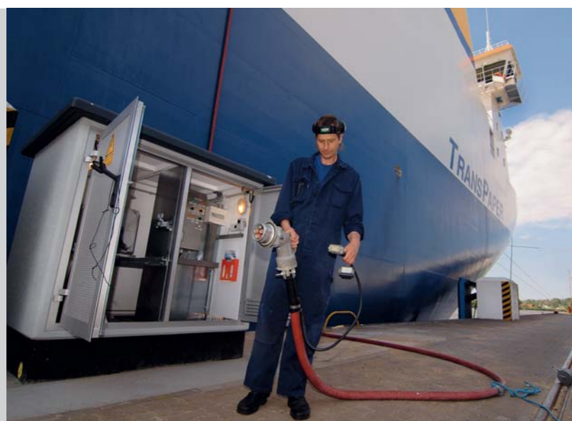
An engineer connects a ship to the onshore power plant.
