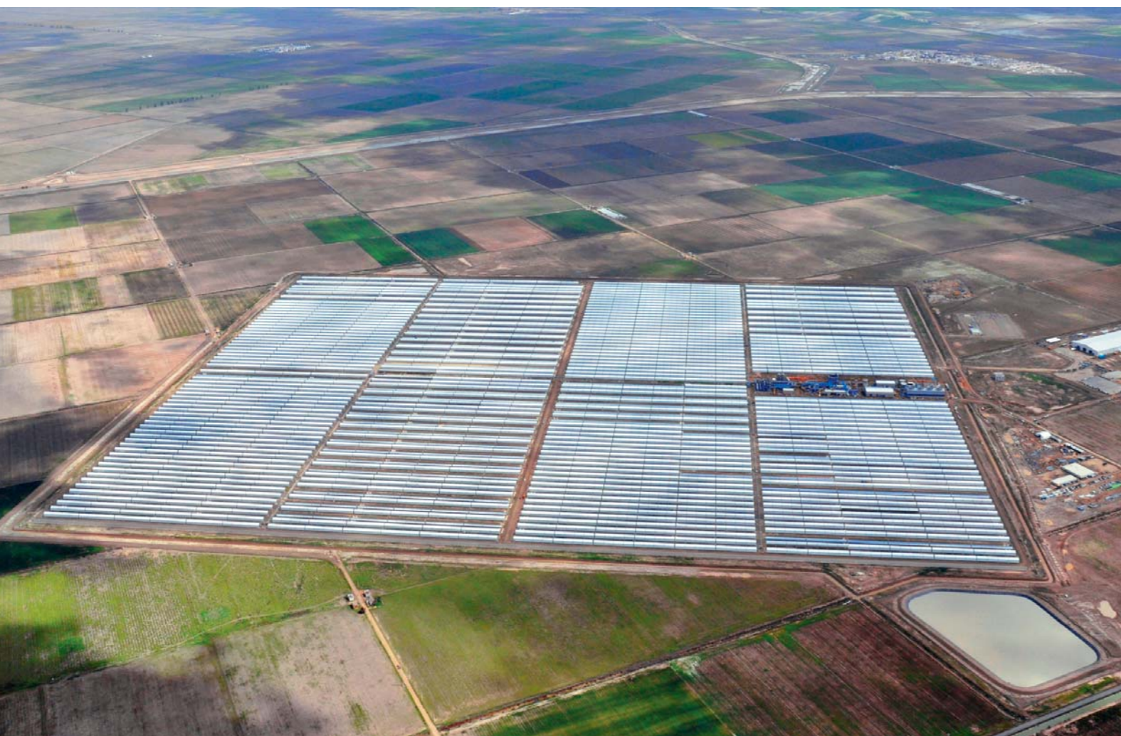
The parabolic troughs at Lebrija, placed side by side, would extend 60 kilometers. Larger plants could operate even more efficiently by making better use of the power plant unit.
