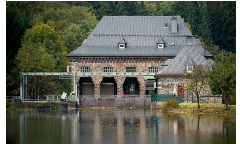
On the exterior, this power station has not changed much since its construction.
