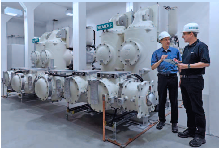
The 8DN8 enhanced gas-insulated switchgear in Kassel.
