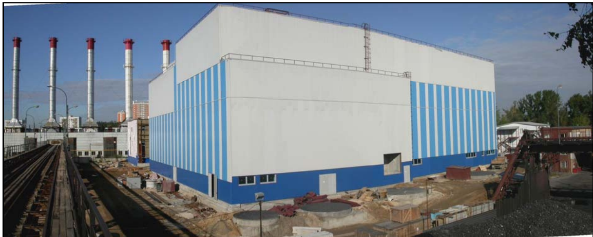
Fig. 3, Phase One is in an advanced stage of completion
