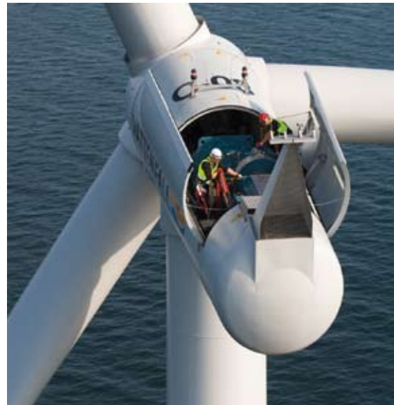
Service technicians at work on an SWT-2.3-93
