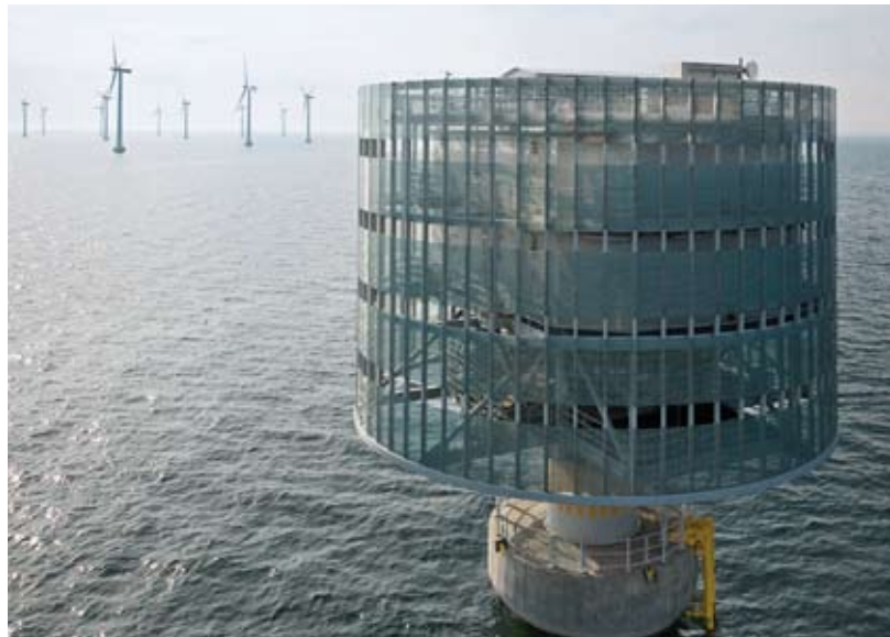
Siemens can also supply turnkey grid connections for wind farms, including construction of the offshore transformer station
