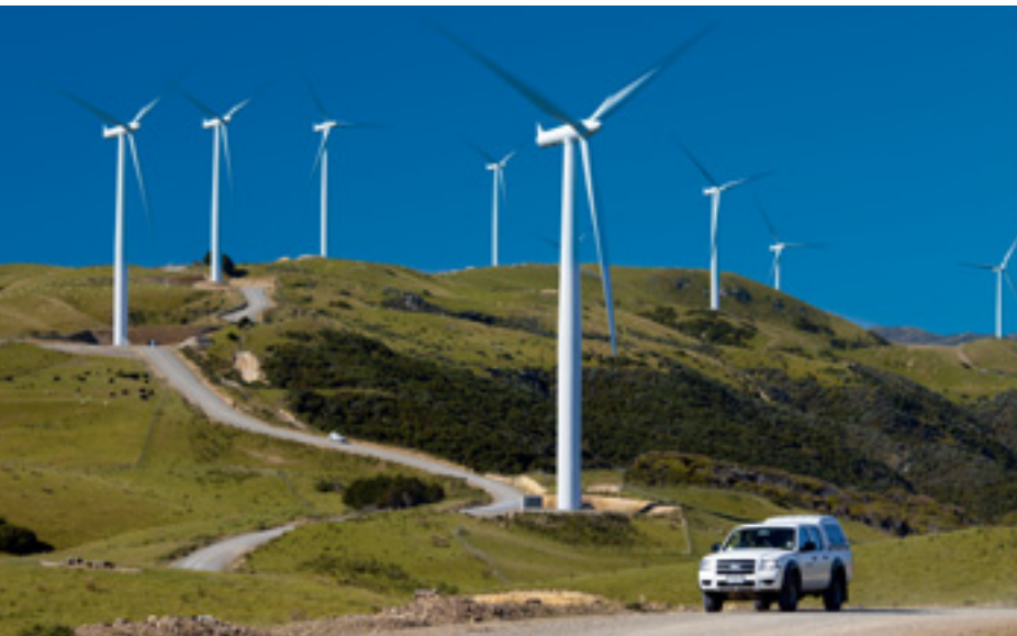
At West Wind, New Zealand, Siemens supplies one-stop solutions and a comprehensive range of services for onshore wind power generation
