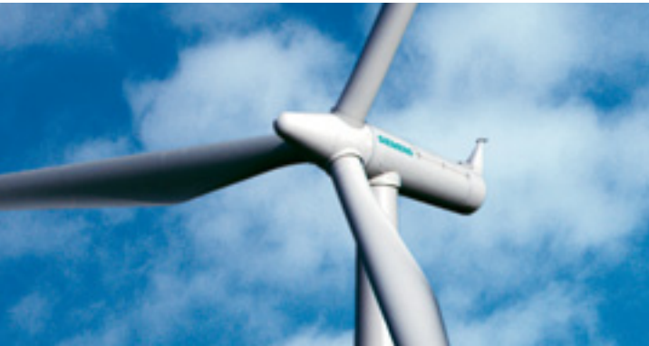
SWT-2.3 wind turbines
