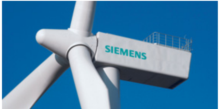
SWT-3.6 wind turbines
