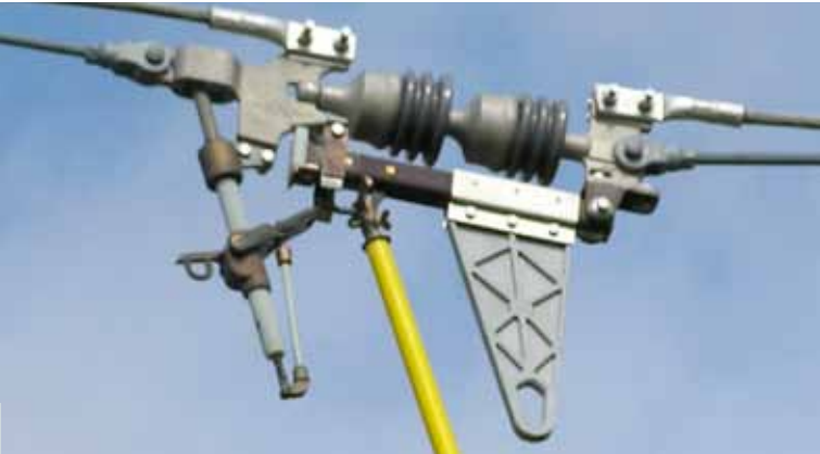
Pull the switch to open via the pull ring...
