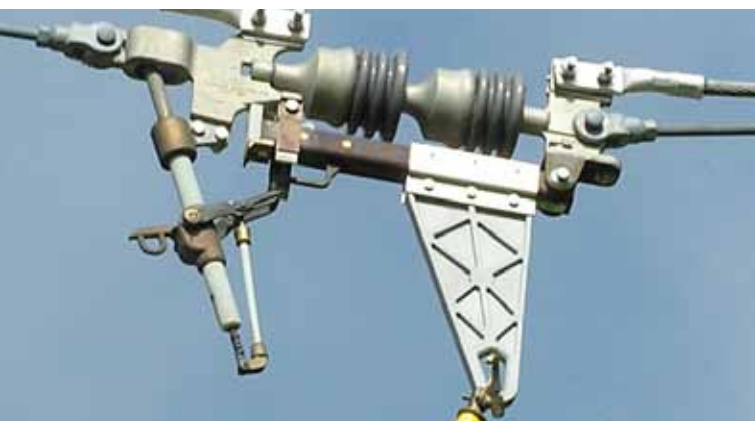
Pull the switch to close via the closer arm...
