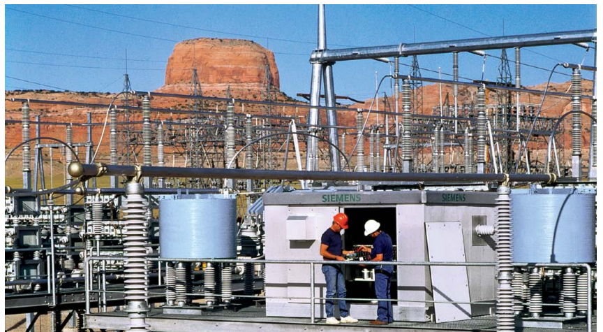
Siemens field technicians at the Kayenta substation.
