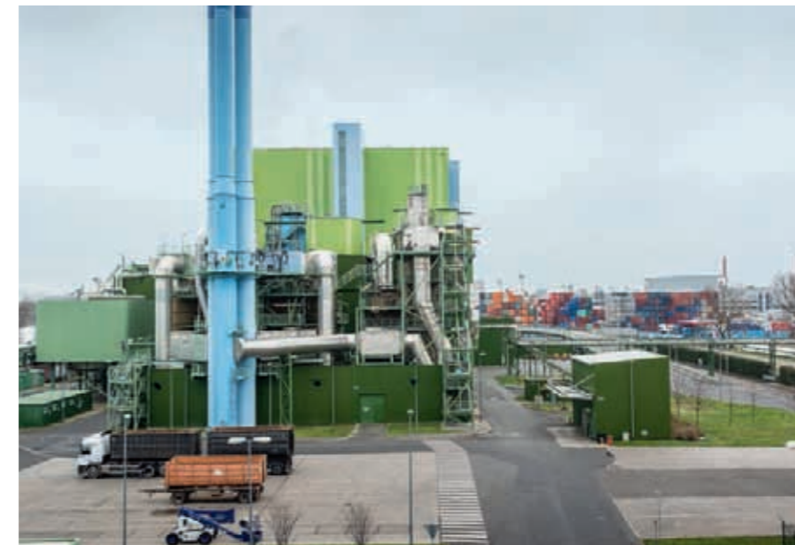
Residual steam from this waste burning facility near the KMW plant will soon be used to maintain KMW's hot-start capability.
