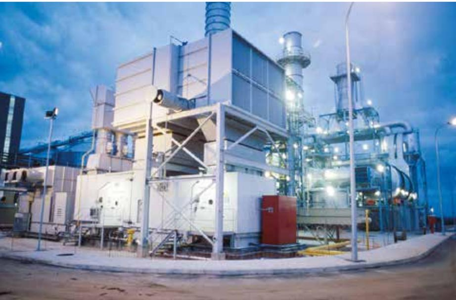
*“Each DLE canister combustor can be removed individually in less than an hour for inspection or repair without removing the engine from its berth.”*
