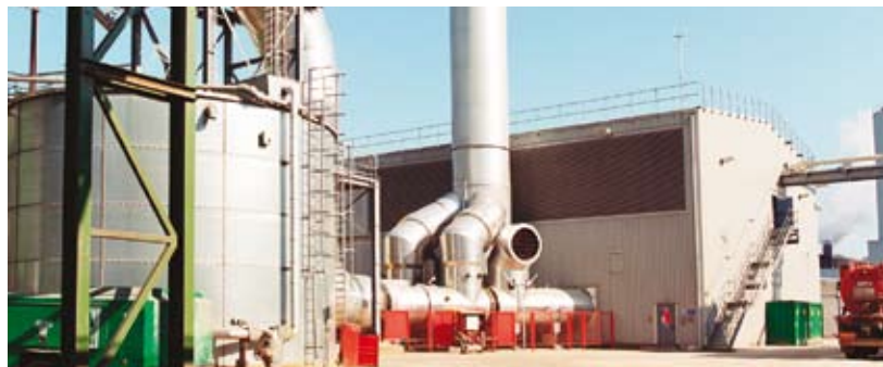
Two SGT-300 gas turbines provide Norbord with electricity and heat at their board manufacturing plant in Scotland, UK.
