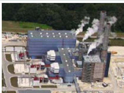
Figure 7. The 860 MW Irsching 5 combined cycle plant (SCC5-4000F 2+1)
